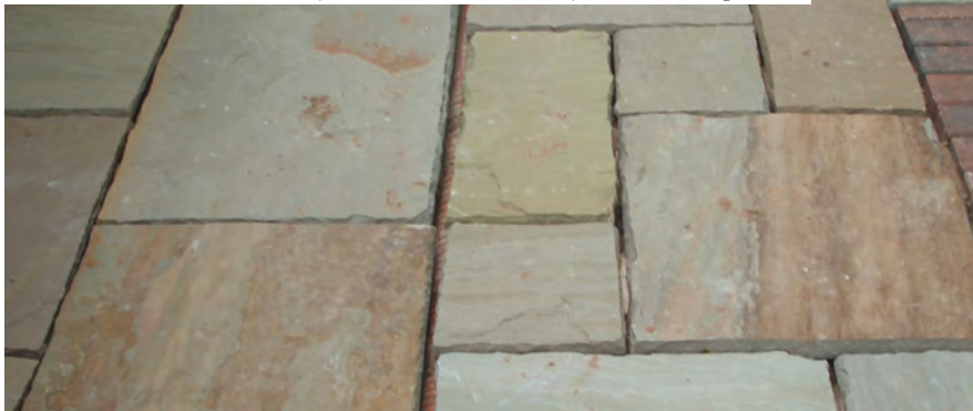
Calibration marks – the straight lines which run across the slabs seen here are on the bottom of the slab and should be laid down
