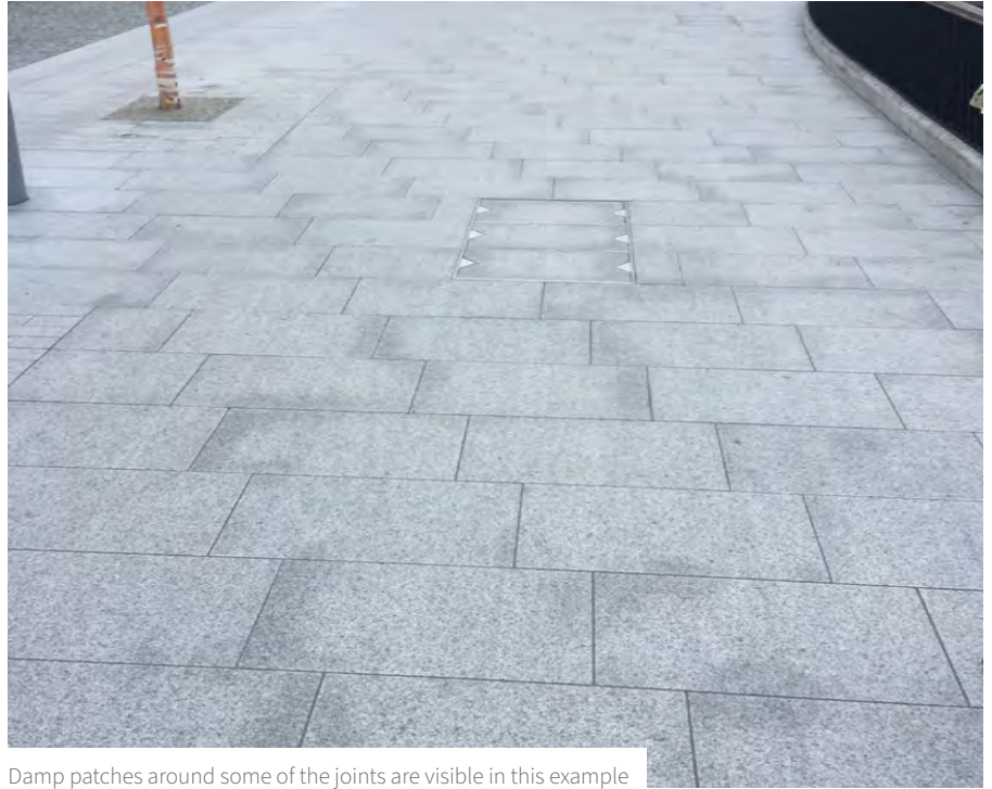
Damp patches around some of the joints are visible in this example
