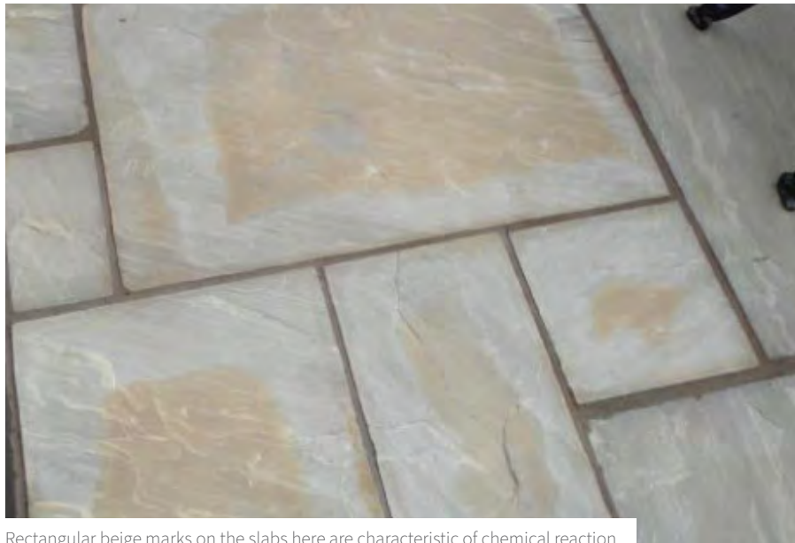
Rectangular beige marks on the slabs here are characteristic of chemical reaction
