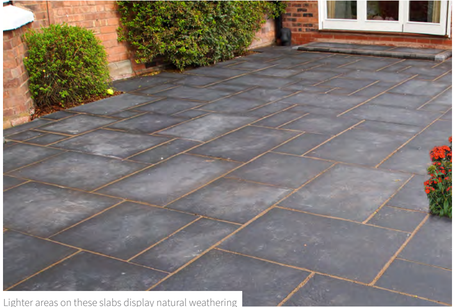
Lighter areas on these slabs display natural weathering
